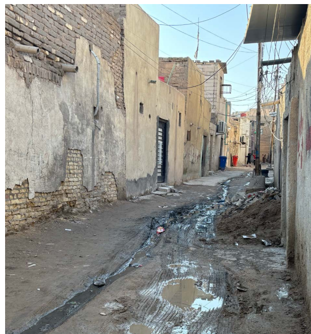
An unpaved side street after a light rain in Zubayr, Iraq.
